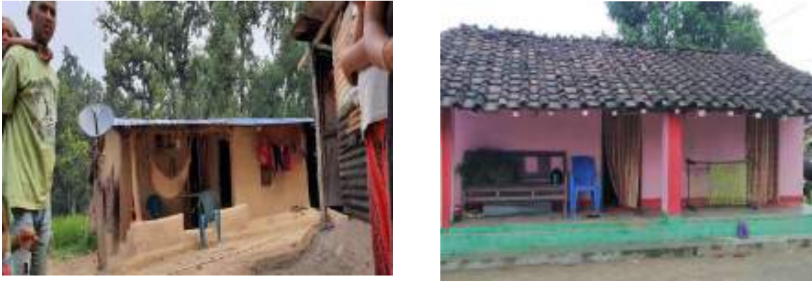
Fig. 4.8 Most vulnerable rural houses during windstorm risk.
