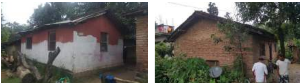
Fig. 3.87 Typical Load Bearing Residential Buildings with CGI & Tiled Roof, Godawari Municipality.
