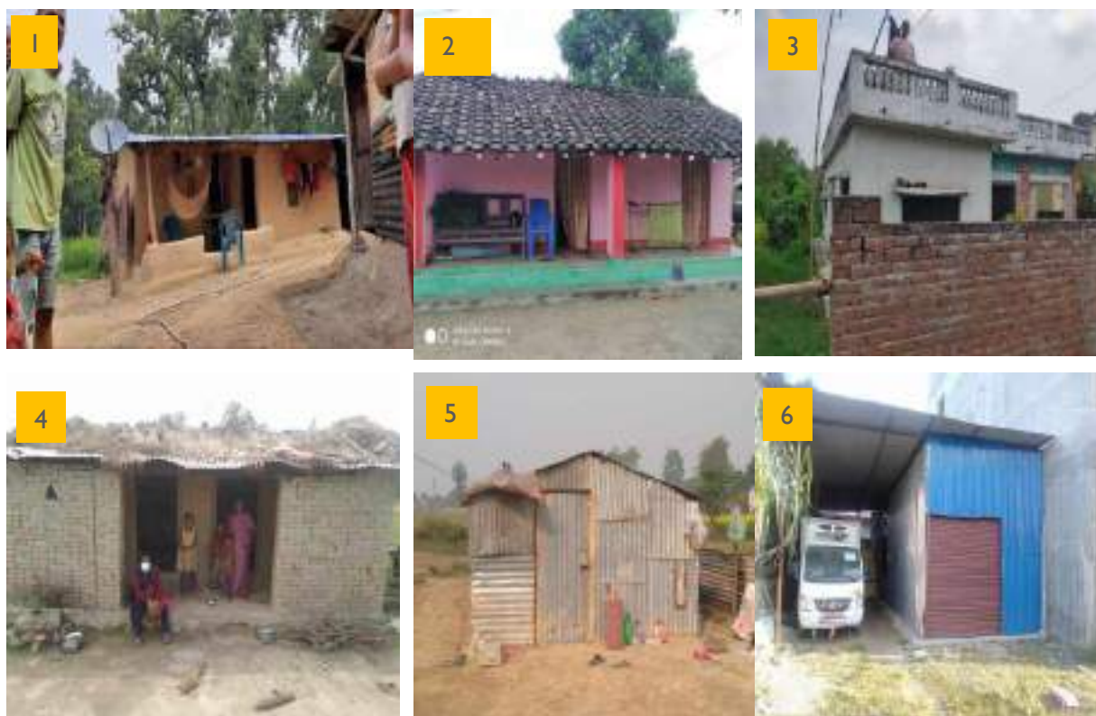
Fig. 3.65 Types of buildings based on the construction type (1: BMW, 2: LBC, 3: RCC, 4: LBM, 5: OTH).
