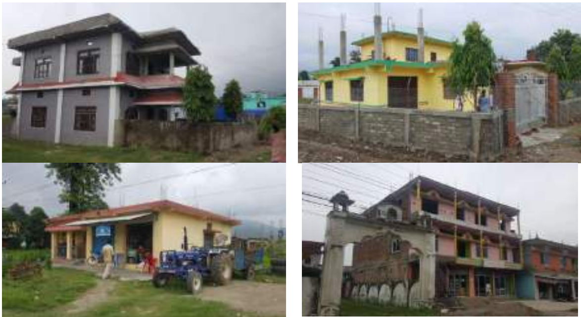
Fig. 3.86 Typical RCC Residential Buildings, Godawari Municipality.
