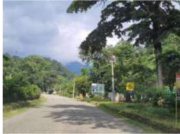
Fig. 2.2 Dhangadhi Highway Black Topped Road connecting from Attariya to Dadeldhura.
