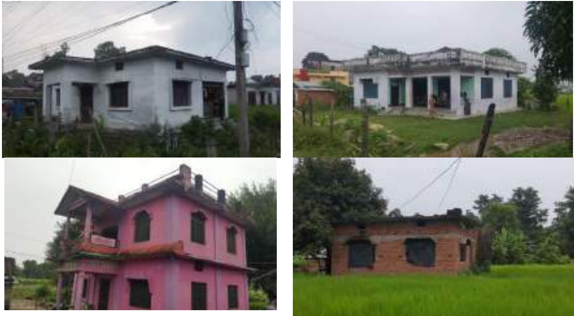
Fig. 3.85 Typical Masonry Load Bearing Residential Buildings, Godawari Municipality.
